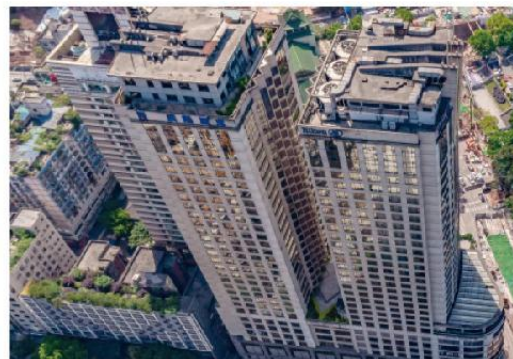
重庆市希尔顿商务楼公区 Public Area of Chongqing City Hilton Commercial Building
