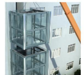
整体吊装 Integral lifting
